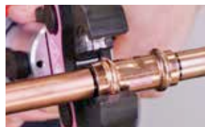
9. Align jaws squarely on the fitting
