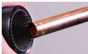
2. Deburr and remove all external sharp edges
