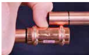
7b. Check the depth mark
